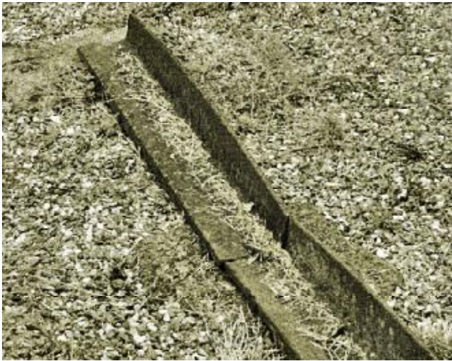
Two pieces of L-shaped cast-iron plate rails, mounted on stone sleeper blocks, originally from the Croydon, Merstham & Godstone iron Railway
