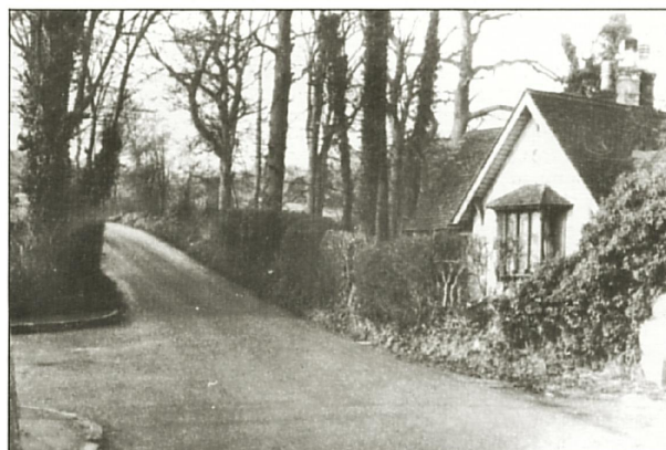
South Lodge: It was removed to make way for widening of Burntwood Lane.
